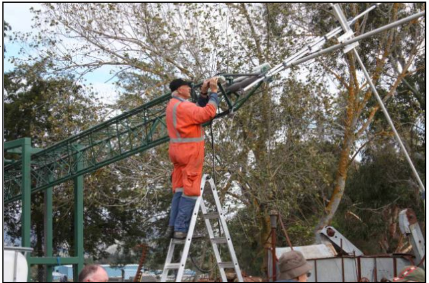
Paul aligning the radios on the tower
