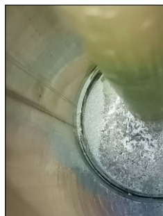
Corrosion inside cavity
