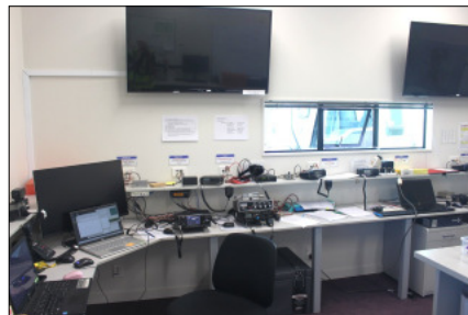
EOC radio room with (L-R) Winlink/VarAC HF, VHF720, DMR, VHF Simplex, VHF695
